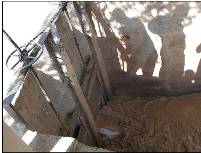
Picture 7: Original intake constructed in the late 1970's
