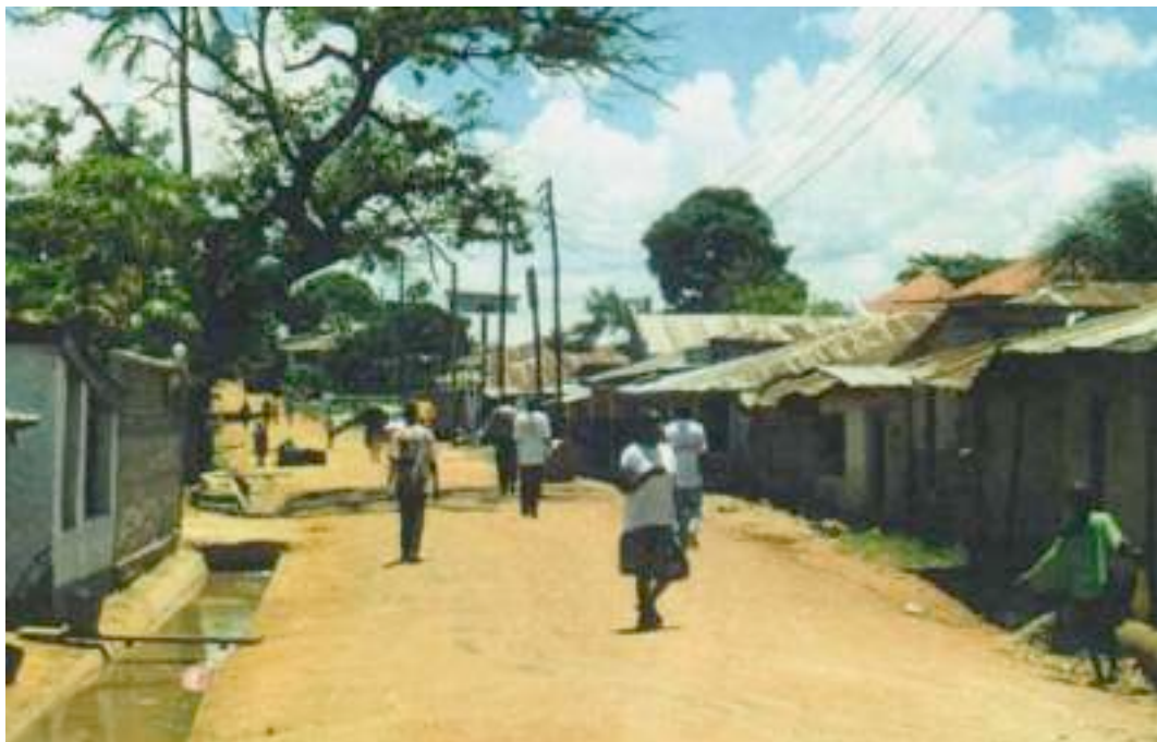
Completed murram roads and side drains. Side drains show lack of maintenance
