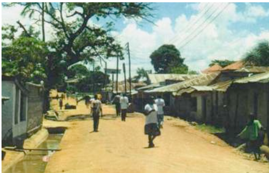
Completed murram roads and side drains. Side drains show lack of maintenance
